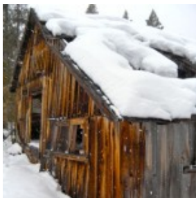
Celio dairy barn in Washoe Meadow State Park.
