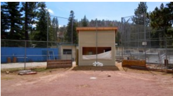
The softball field under construction at STHS.
