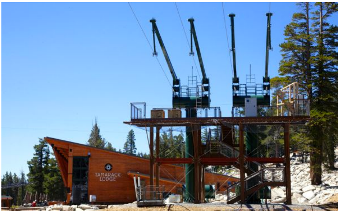
The four-line zipline being built near Tamarack Lodge
