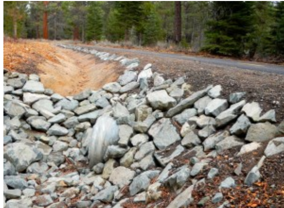
Erosion control measures line the trail.
