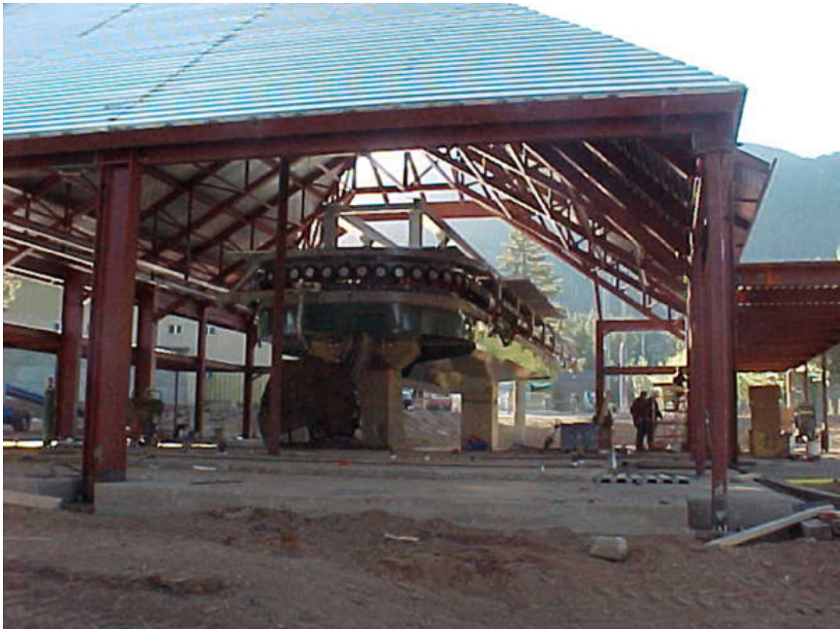
The gondola under construction. Photo/Heavenly Mountain Resort
