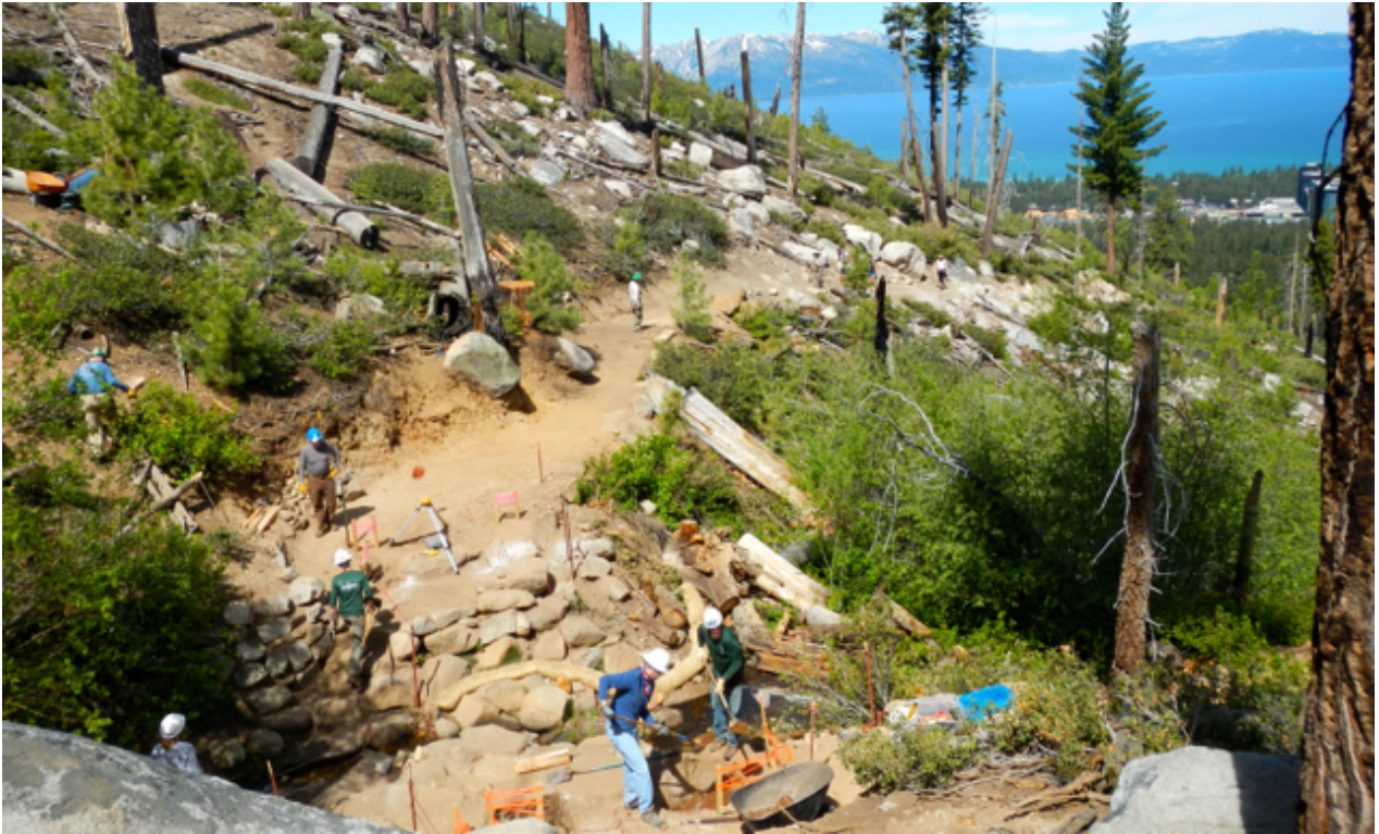
Tahoe Rim Trail volunteers prep the site for a bridge in Van Sickle Bi-State Park. Photo/Kathryn Reed
