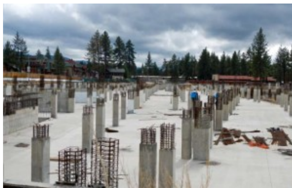
Work on the hole could begin
