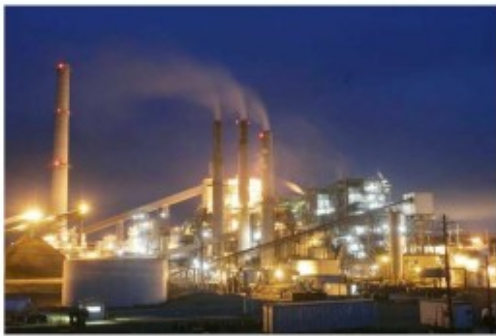
The coal-fired Reid Gardner Generating Station near Moapa. Photo/Sam Morris/Las Vegas Sun
