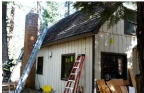
A fire in Tahoe Vista was damaged by fire Sept. 25. Photo/Provided
