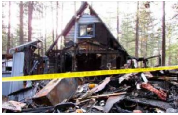
Not much could be salvaged from this house after it burned in January. Photo/Denise Haerr
