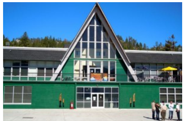
Lake Tahoe Airport doubles as city hall.
