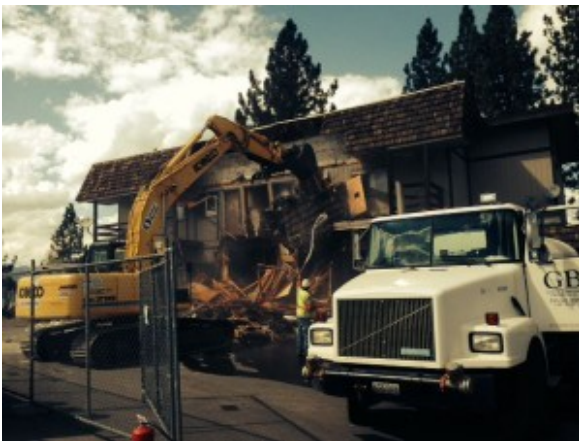
The building being razed Sept. 15. Photo/Provided
