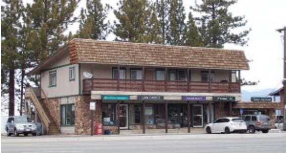
The Alta Mira building. Photo/Bill Kingman
