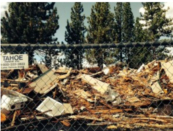
The pile of debris.
