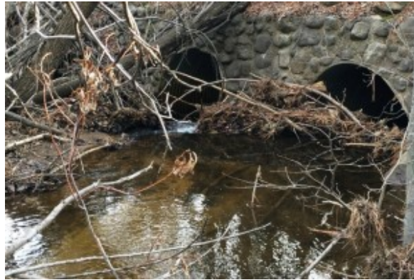
Improvements to Incline Creek should be finalized this year. Photo/Provided
