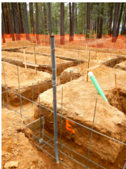
Underground utilities are in place at the animal cages.
