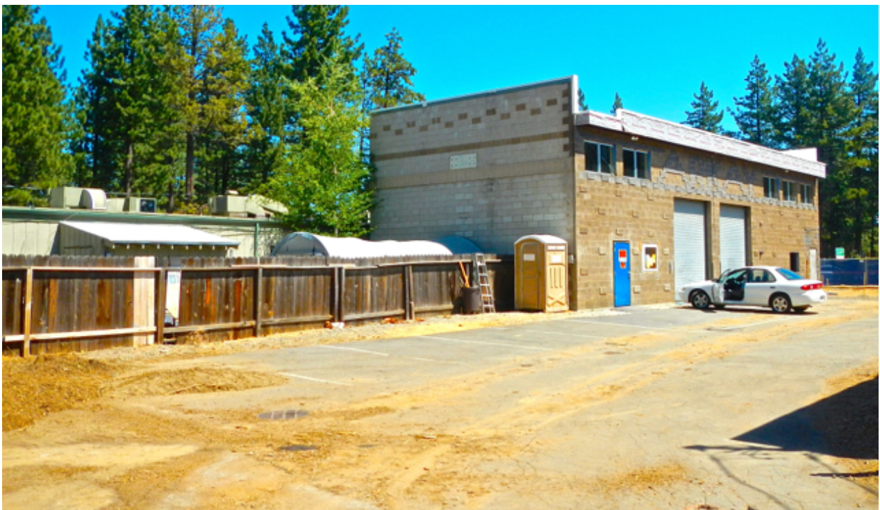
Additional commercial floor area was acquired at Harrison Avenue to create a rooftop dining area. Photo/LTN
