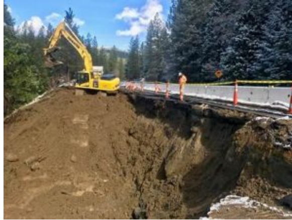
Crews use a break in storms to work on Highway 50 by Bridal Veil falls. Photo/Caltrans
