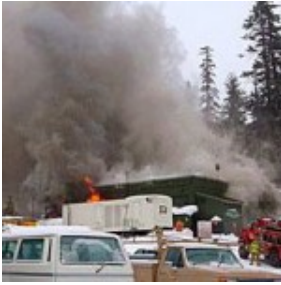
Kirkwood's power plant goes up in flames Jan. 1. Photo/News 10- ABC
