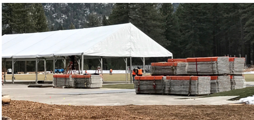
A protective layer is being placed on the South Lake Tahoe ball field. Photo/LTN
