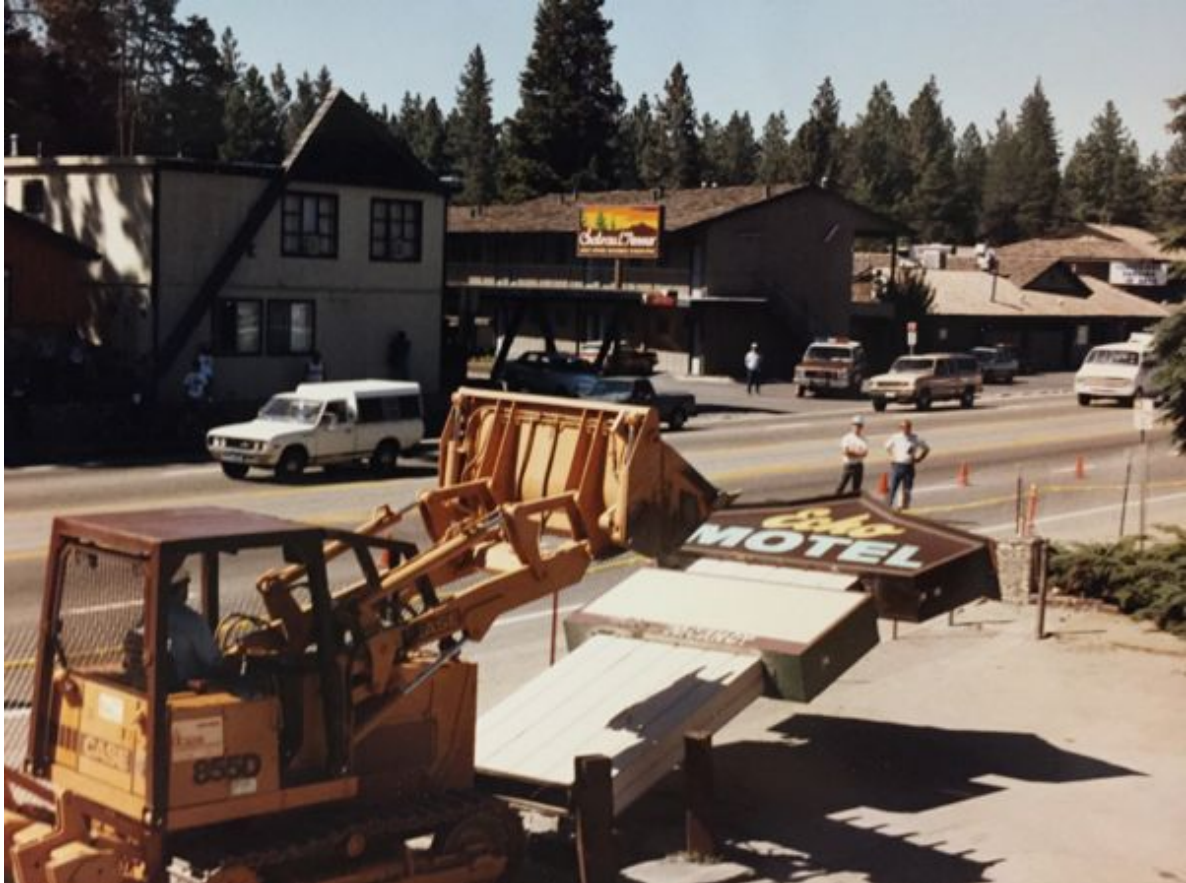
Echo Motel on Highway 50 and Ski Run Boulevard comes down June 26, 1989, for the first phase of redevelopment. Photo/South Lake Tahoe
