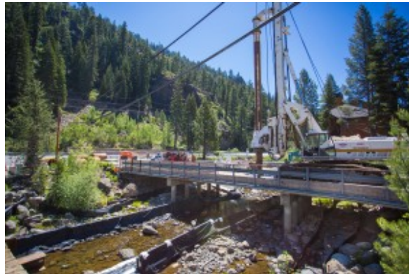
Alpine Meadows Bridge replacement. Photo/Erik Bergen
