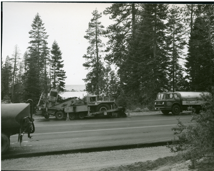
Paving of Highway 28 in August 1985. Photo/NDOT
