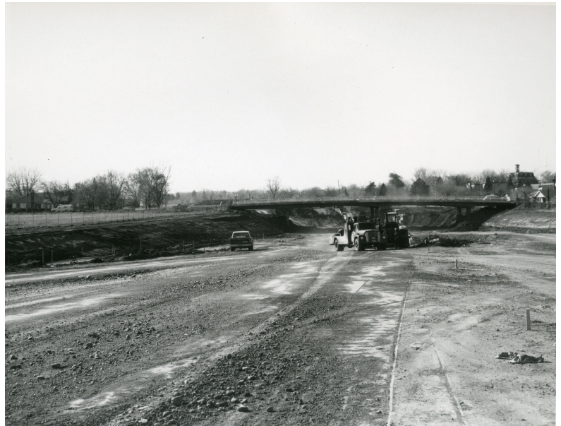
Building Interstate 80 near Reno in May 1972. Photo/NDOT
