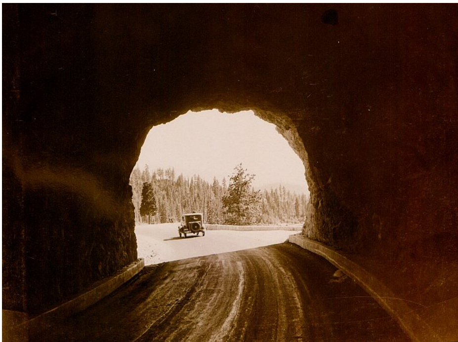
Cave Rock tunnel, circa 1930s. Photo/NDOT
