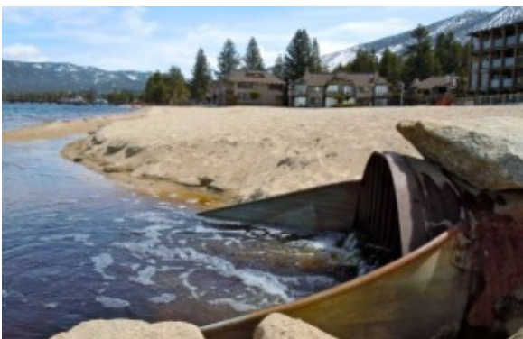
This storm pipe near Lakeshore Lodge and Spa in
