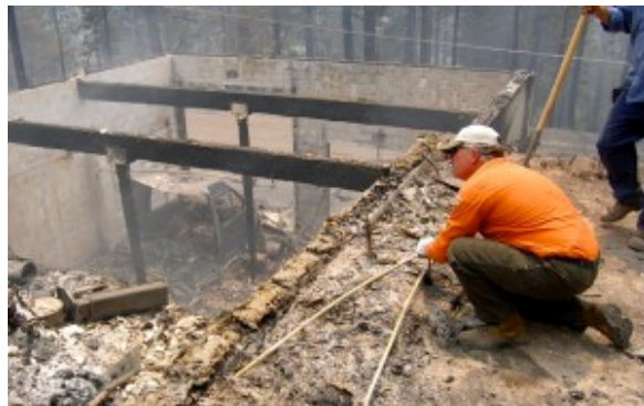
South Tahoe PUD crews crip water supply lines in the Angora burn area. Photo/STPUD
