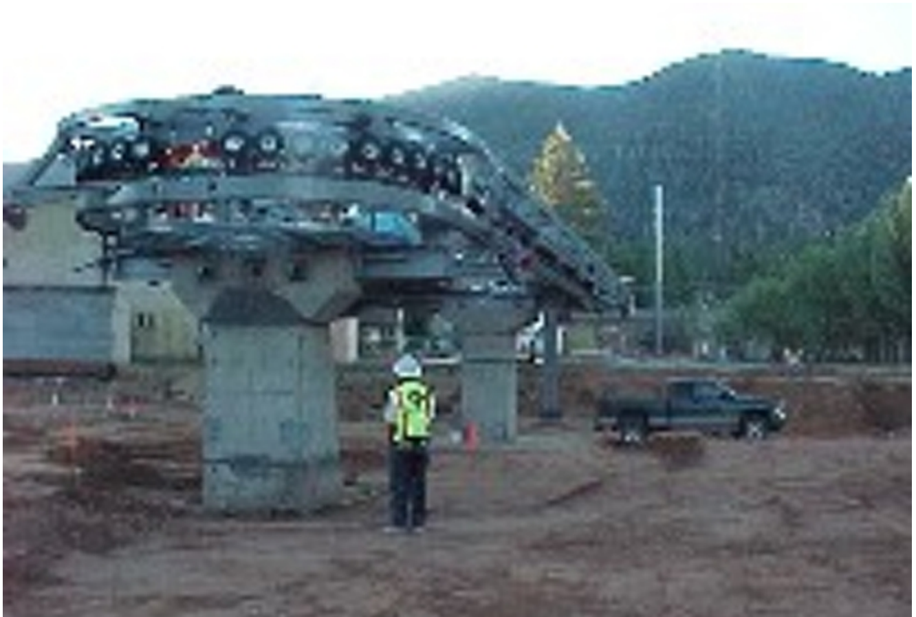
The base of the gondola was put in by American Ski Company. Photo/Heavenly Mountain Resort
