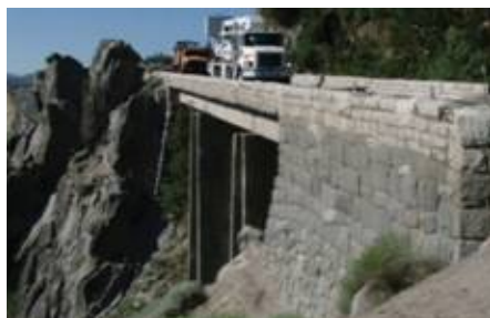
Caltrans plans to replace this Echo Summit bridge in 2019. Photo/Provided
