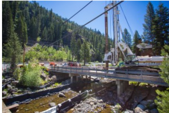
Alpine Meadows Bridge replacement. Photo/Erik Bergen
