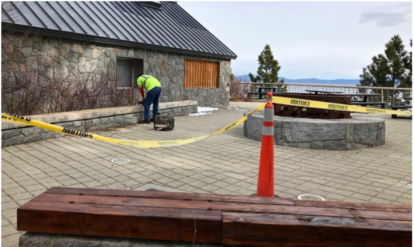
A South Lake Tahoe employee works to get Lakeview Commons spruced up for the summer season. Photo/Kathryn Reed
