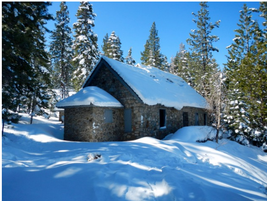
The structures at Skunk Harbor are not open to the public. Photo/Kathryn Reed
