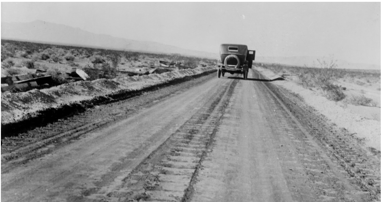
A completed sand and oil surface except for the final dragging, circa 1919. Photo/NDOT
