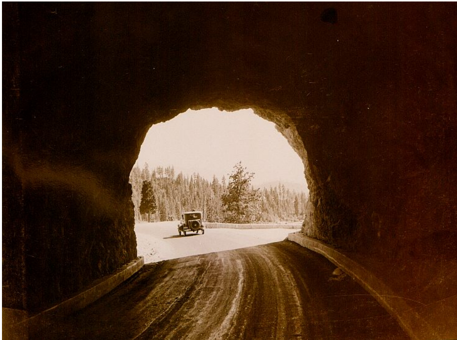
Cave Rock tunnel, circa 1930s. Photo/NDOT
