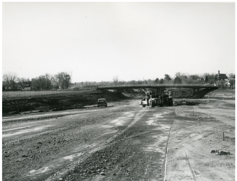
Building Interstate 80 near Reno in May 1972. Photo/NDOT
