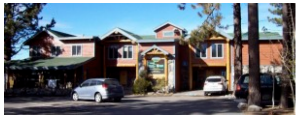
The Lake Front Building today.
