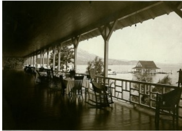
View from the Baldwin estate.
