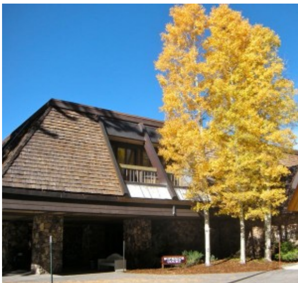
El Dorado County courthouse in South Lake Tahoe needs substantial repairs. Photo/LTN file
