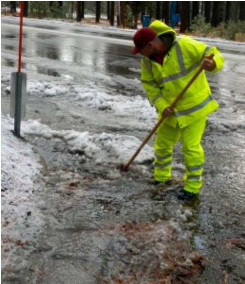
Bobby Maxwell with South Lake Tahoe public works on Nov. 30 clears a storm drain on Ski Run and David. Photos/Kathryn Reed
