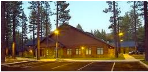
The Juvenile Treatment Center in South Lake Tahoe opened in 2004. Photo/LRS Architects
