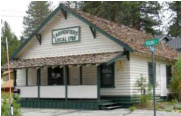
Today the building is used by the carpenters union. Photo/Bill Kingman
