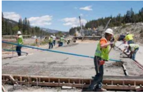
Workers form new concrete on a segment of Interstate 80 near Emigrant Gap and Cisco Grove. Photo/Caltrans
