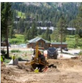
Construction of Kirkwood's
