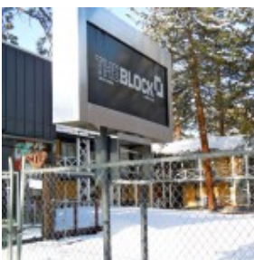
Graffiti and boarded up windows at The Block.
