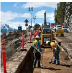
Work on Echo
