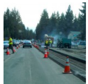
Construction season in South Lake Tahoe.
