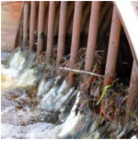
A stormwater drain near the Bijou Center in April 2011. Photo/LTN
