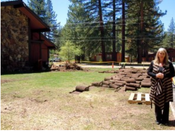
Sharon Bishop is overseeing the renovation of the Barton Community Clinic. Photo/Kathryn Reed
