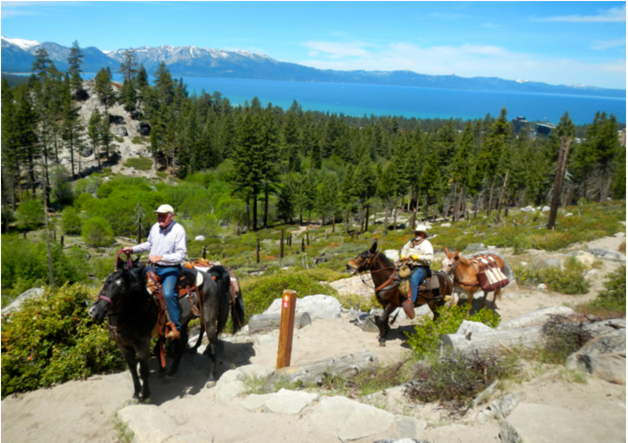
Horses bring the sacks of cement to the worksite. Photo/Kathryn Reed
