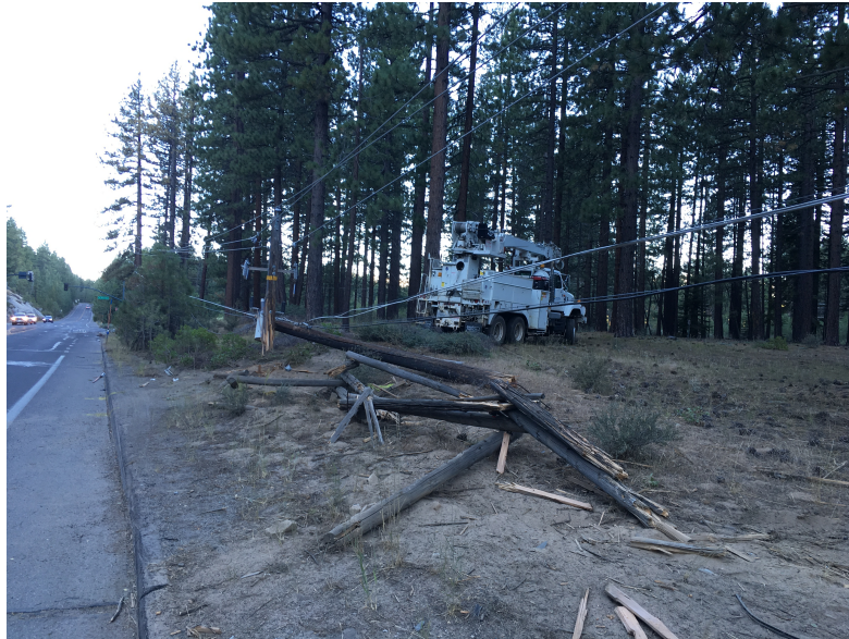
Liberty Utility crews work to repair a splintered power line on Aug. 9. Photo/LTN
