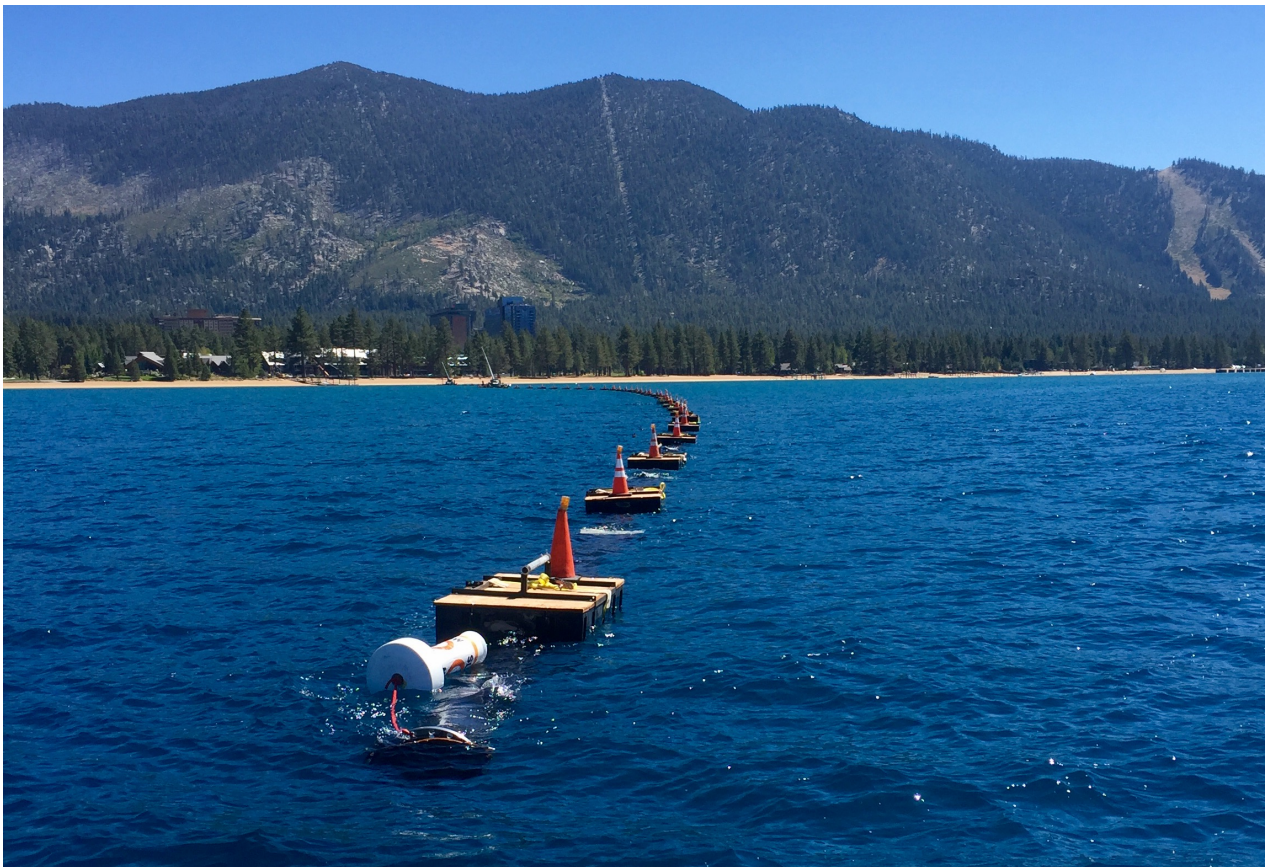
Edgewood Water Company is extending the in-take line 3,000 feet into Lake Tahoe. Photo/LTN
