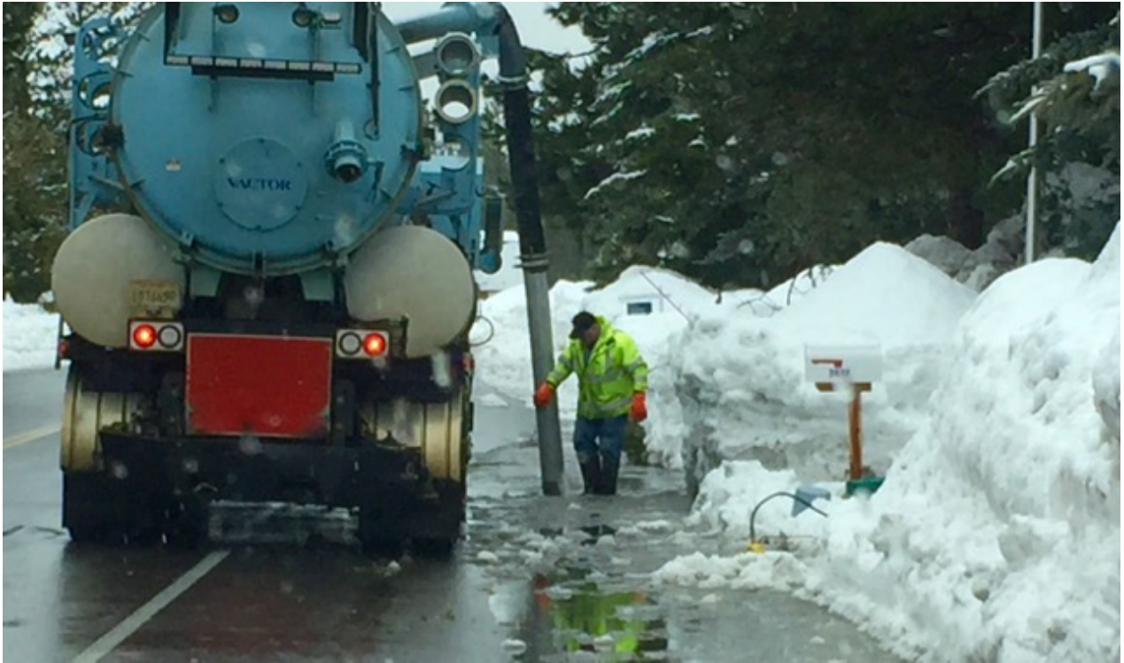
South Lake Tahoe crews on Feb. 10 unclog drains in the city. Photo/Kathryn Reed
