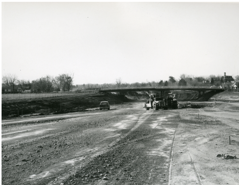
Building Interstate 80 near Reno in May 1972. Photo/NDOT
