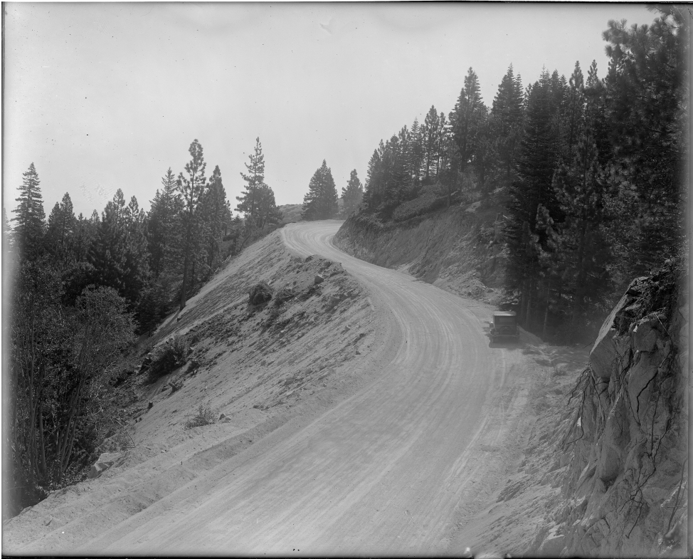
Paving trails through the mountains took special engineering, circa 1920. Photo/NDOT
