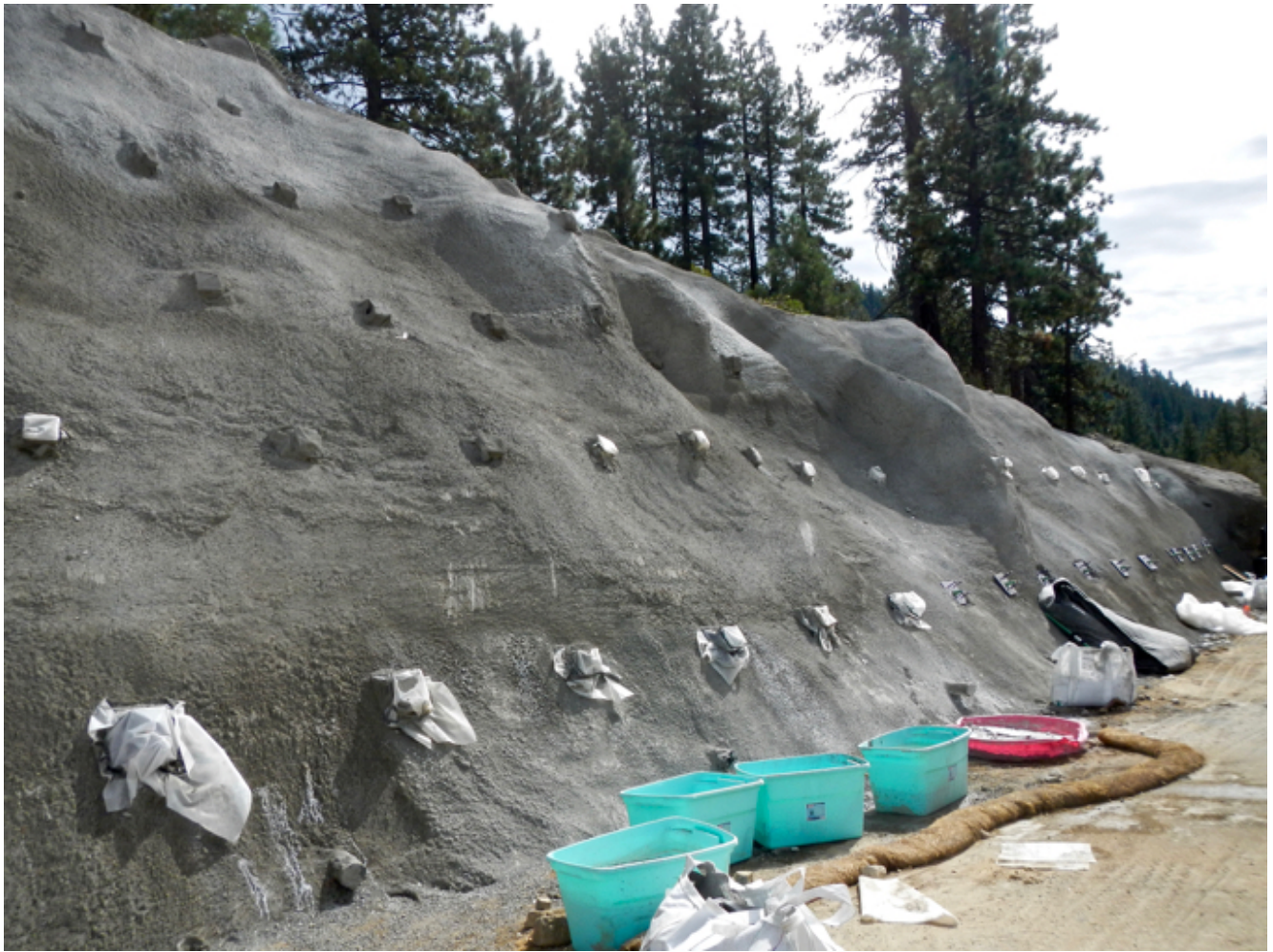
A section of the hillside with the 4-inch concrete spray and limited contouring. Photo/Kathryn Reed
