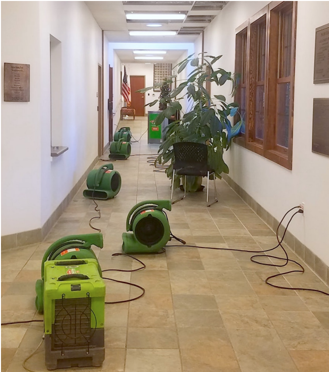
Alpine County administrative offices dry out. Photo/Provided
