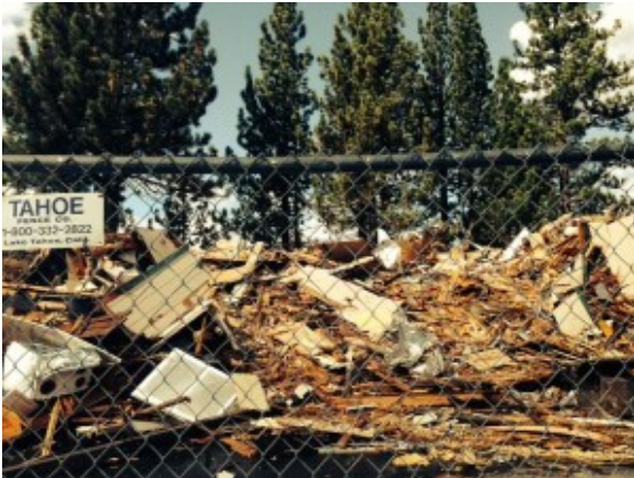
The pile of debris. Photo/Provided
