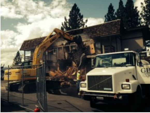
The building being razed Sept. 15. Photo/Provided
