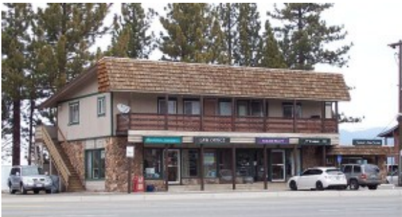
The Alta Mira building. Photo/Bill Kingman
