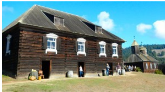
The original buildings still dot the landscape.
